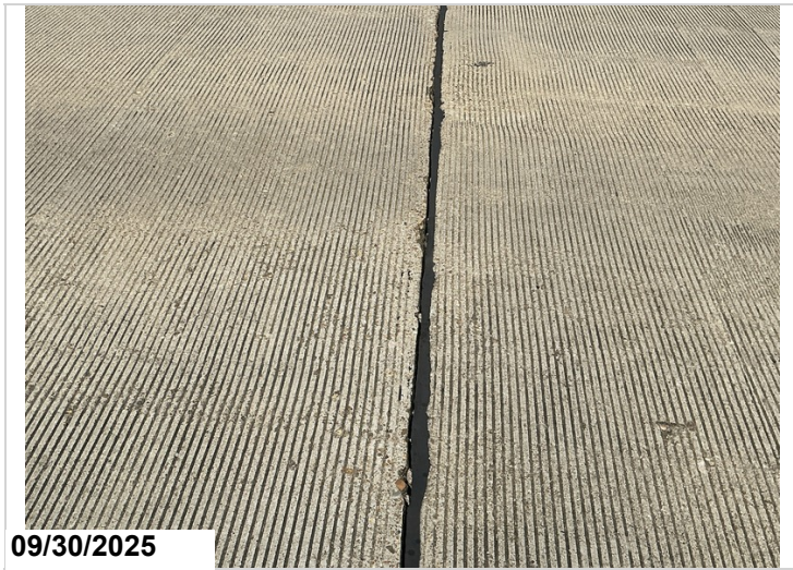
Bent 2 joint, lost adhesion
