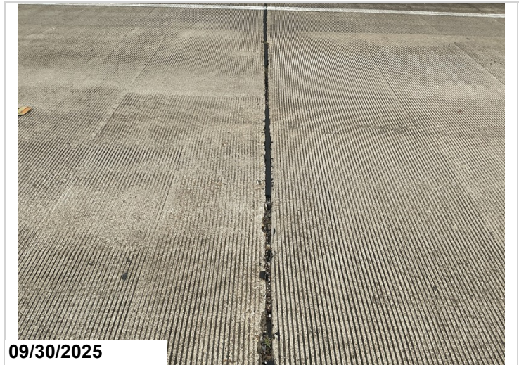
Bent 5 joint missing 6'
