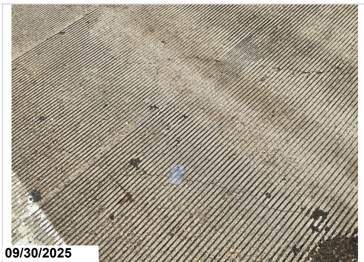
Span 1, diagonal cracks, 0.030.
