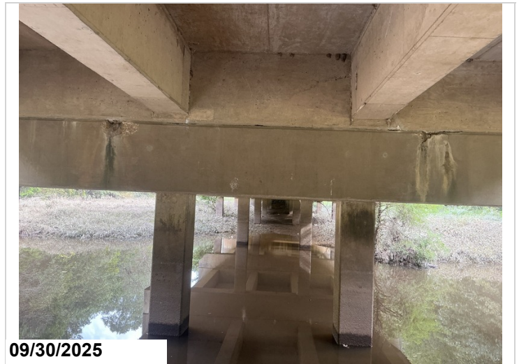
Bent 3 cap back spalls at keyways 2' CS3.
