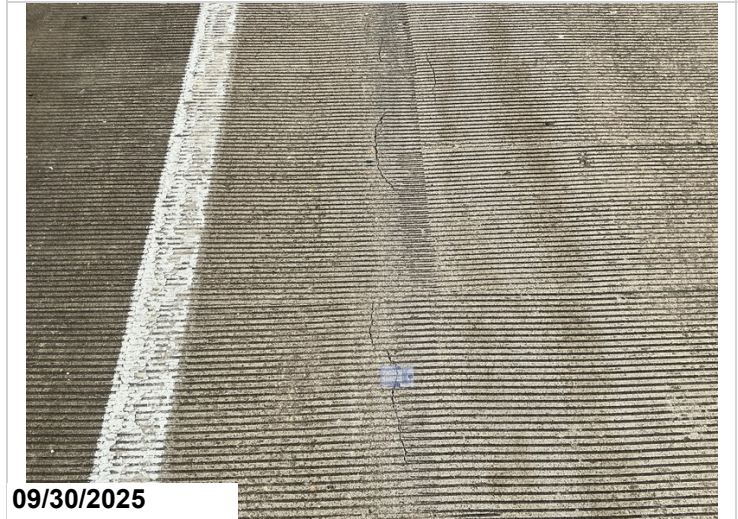
Span 4, longitudinal cracks 0.070 5'
