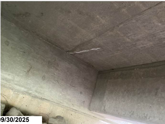
Span 8 bay 3 efflorescence 3' CS2
