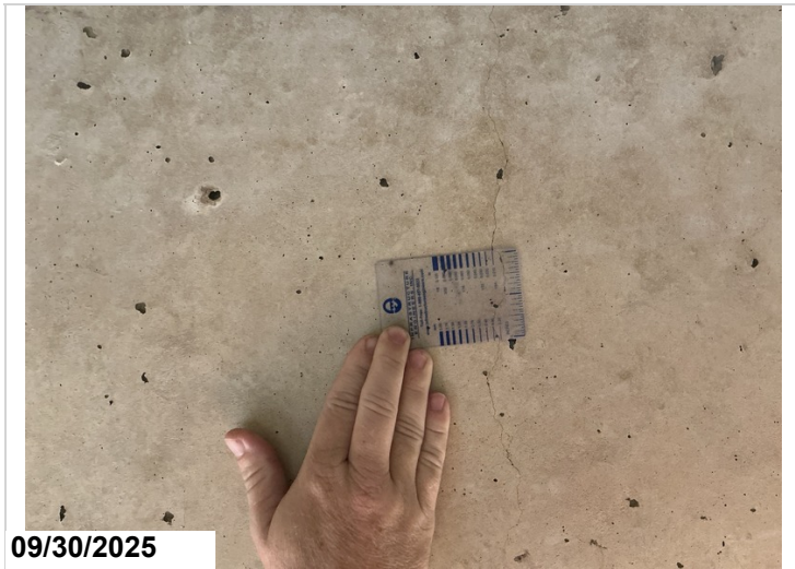
All girders have vertical cracks
